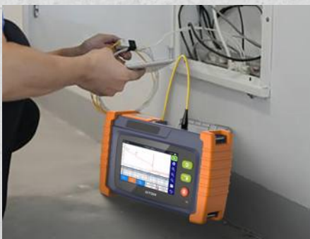
Broadband construction in residential area
