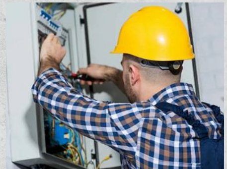
Installation and maintenance works
